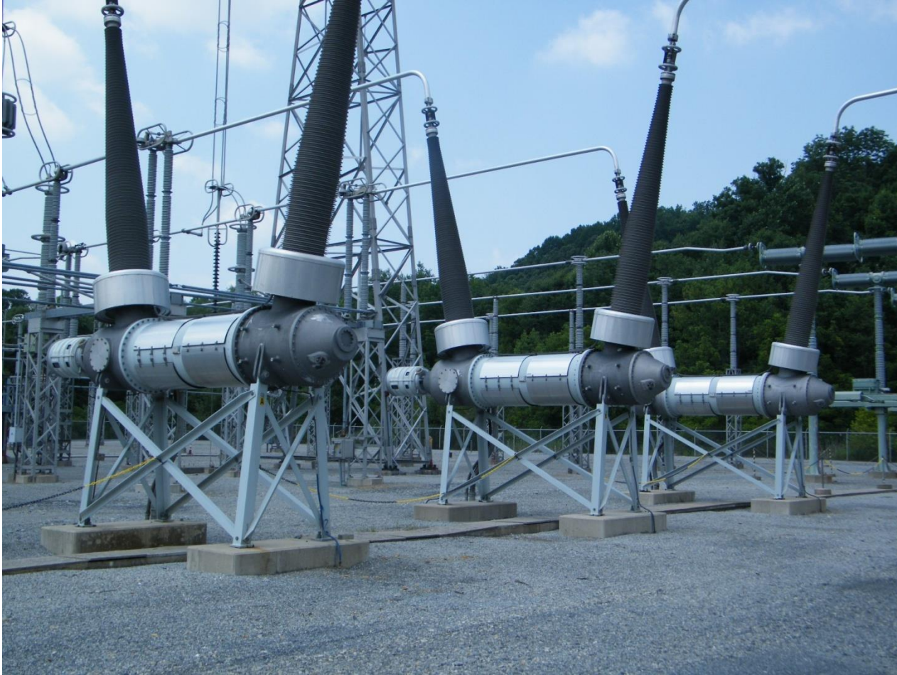
500 kV SF-6 Circuit Breakers
