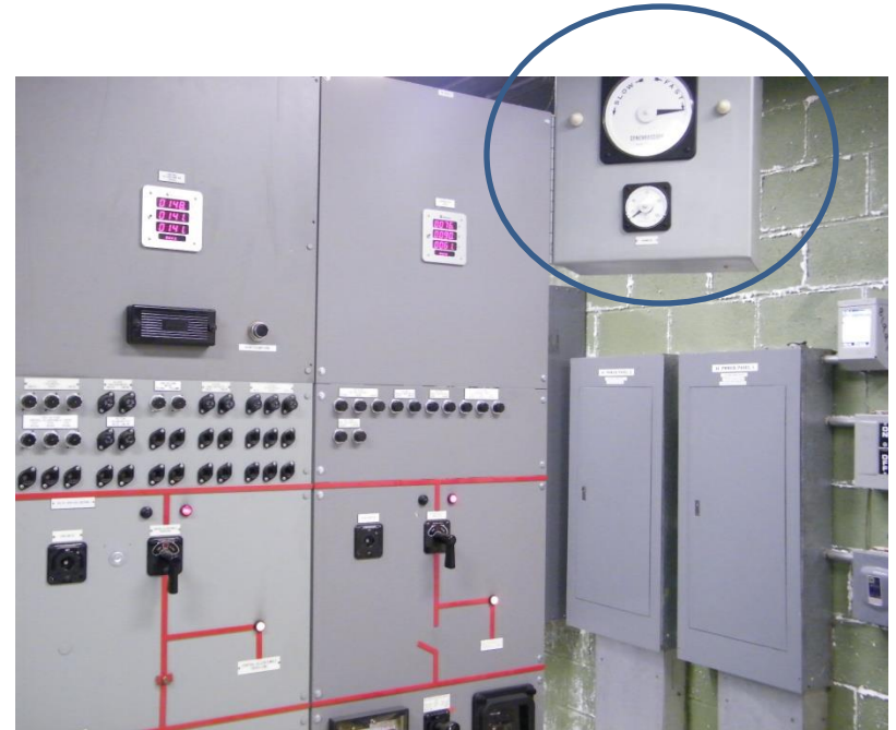
Mimic bus with synchroscope
