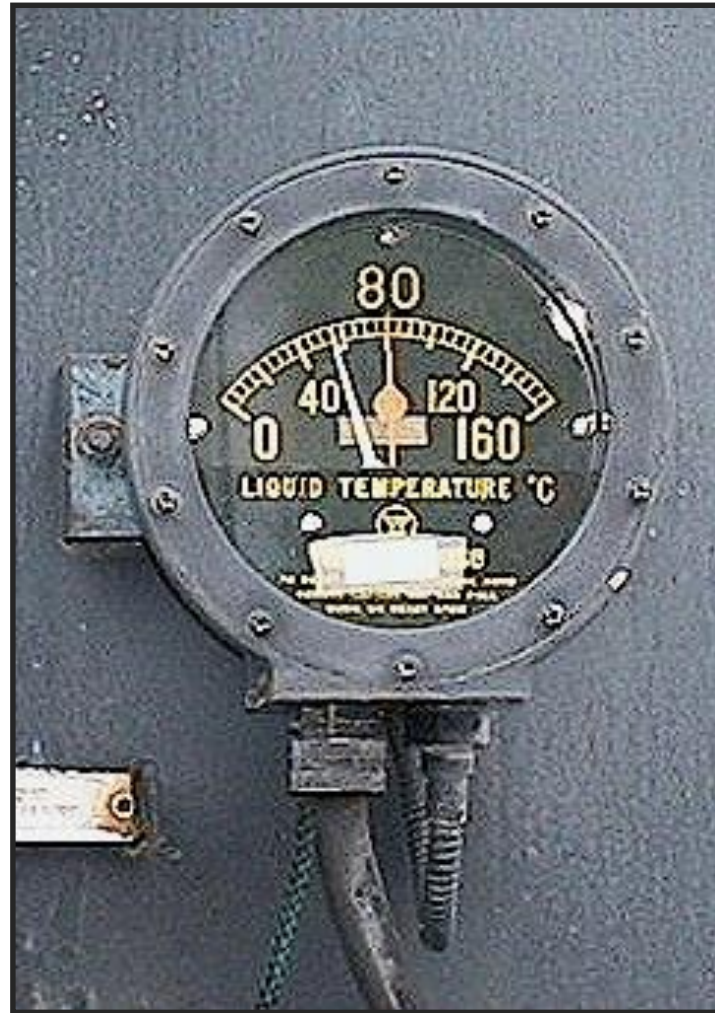
Illustrations of Analog Gauge Style Winding Temperature and Liquid Temperature Thermal Devices
