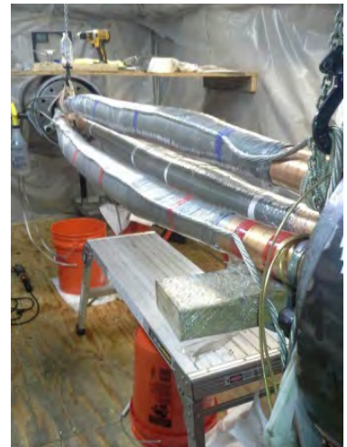
Figure 5- HPFF Repair Splice (provided by BGE)
