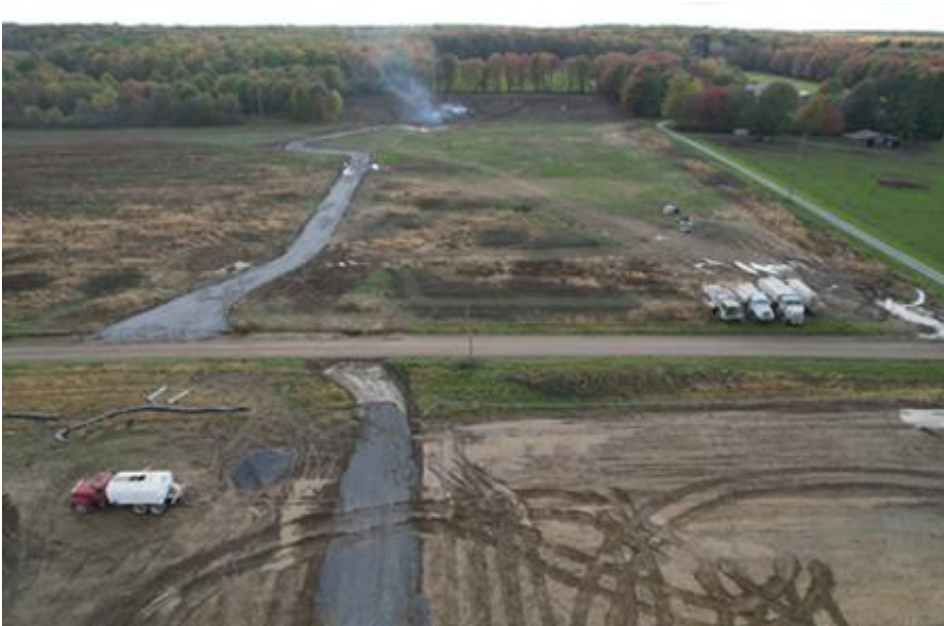
Evidence of Substantial Site Work Provided to Demonstrate Cure (October 16, 2024)
