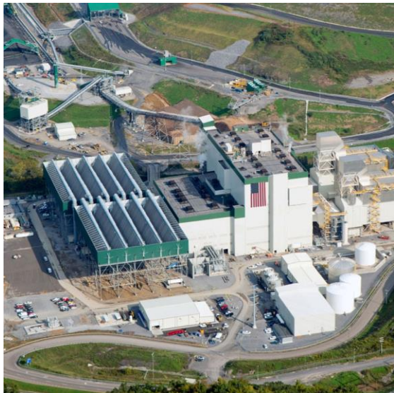
Combined Cycle Generator
