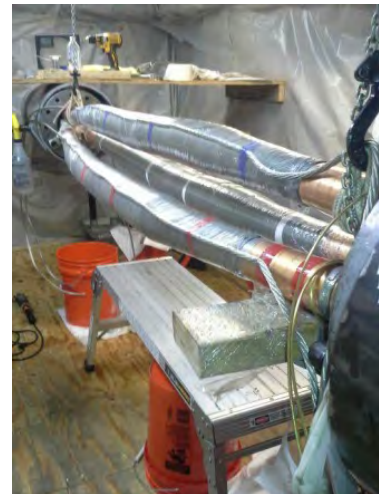
Figure 5- HPFF Repair Splice (provided by BGE)
