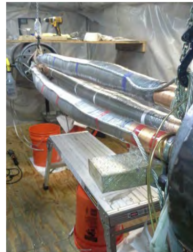
Figure 5- HPFF Repair Splice (provided by BGE)
