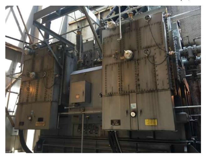
Given the age, condition and layout of the equipment there is concern that a transformer fire or catastrophic failure of other equipment in the station would likely result in the destruction of the whole facility and the loss of 300 MVA of critical load for an extended period of time. Several alternatives were evaluated to address this issue.
