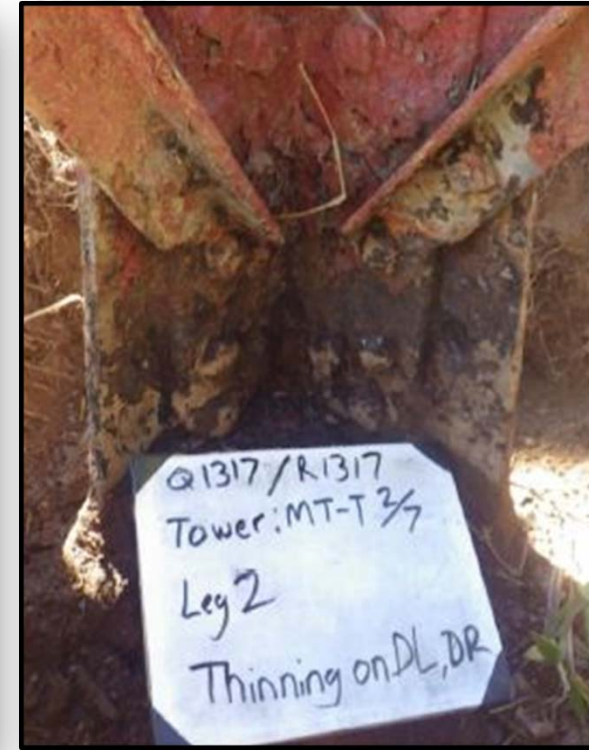
Figure 1: Examples of 25-30% foundation structure loss
