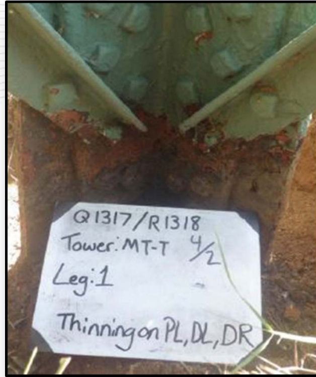
Figure 1: Examples of 25-30% foundation structure loss
