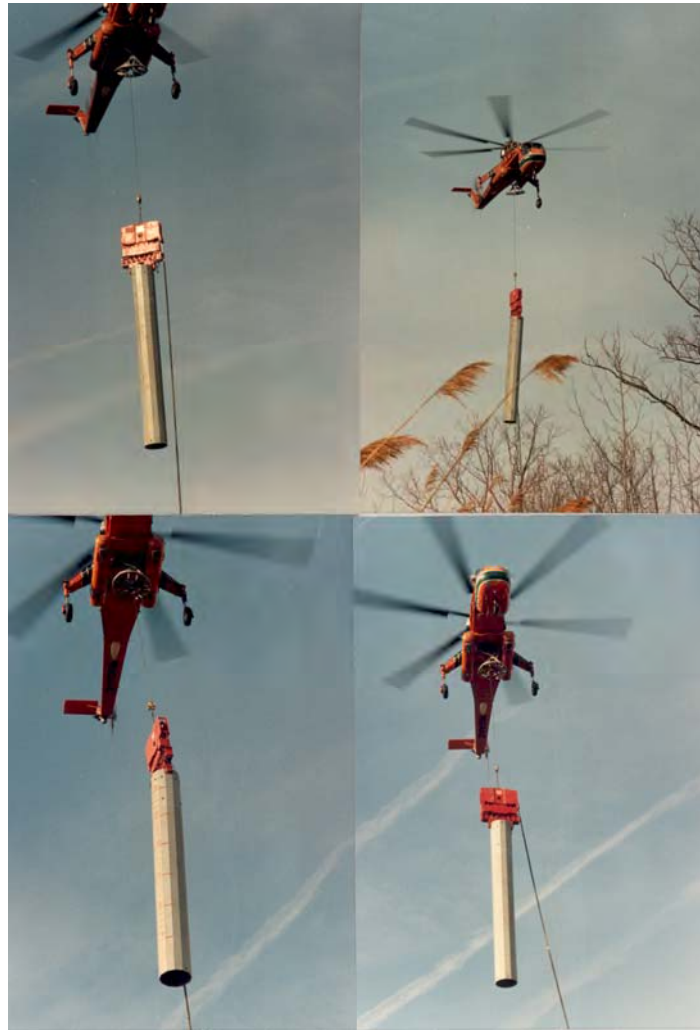
Helicopter Installation of Transmission Pole
