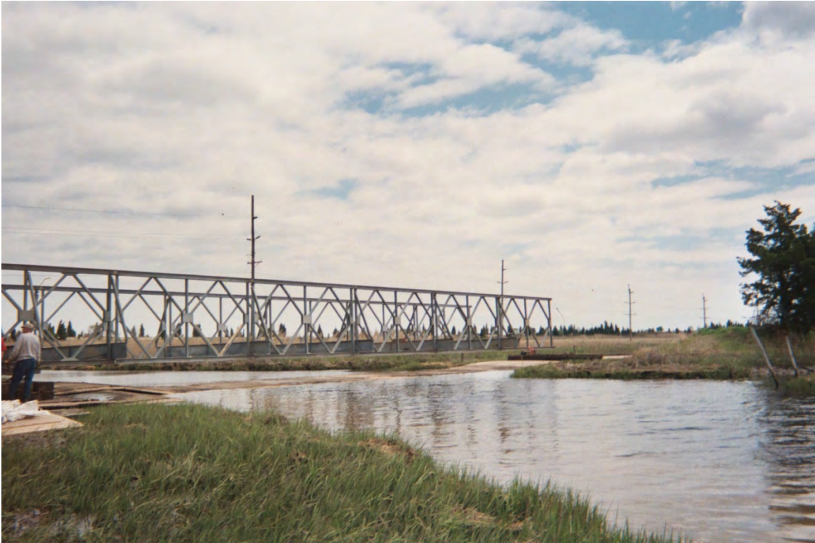
Temporary Bridge Waterway Crossing
