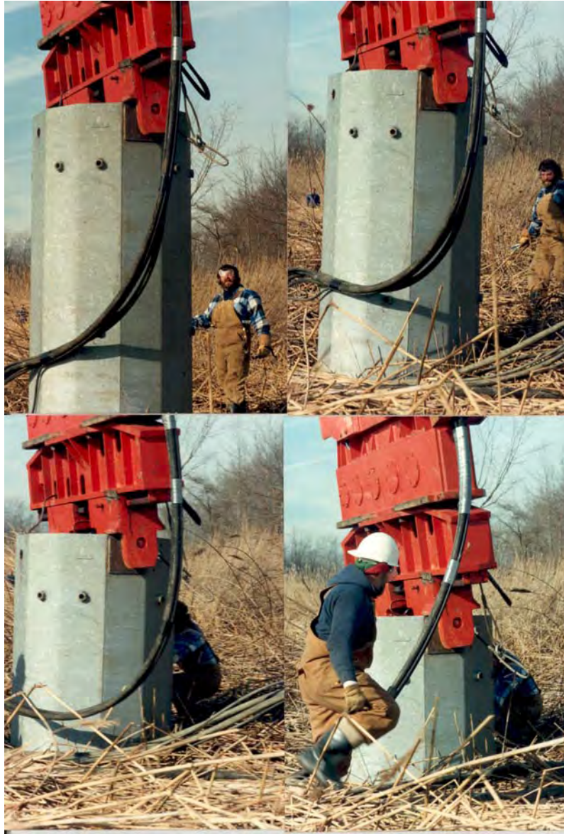
Helicopter Installation of Transmission Line within a Wetland
