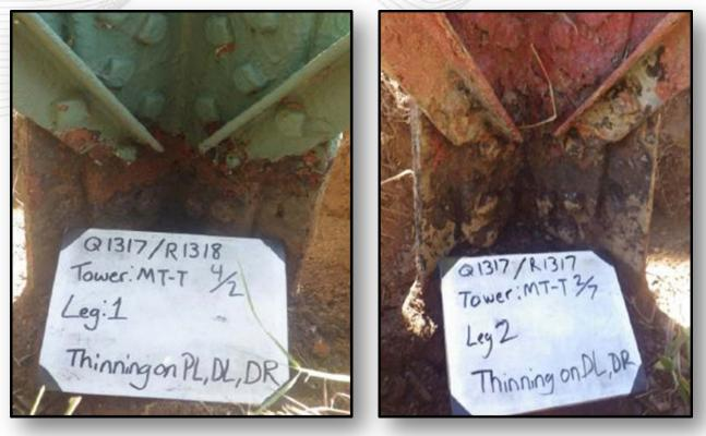
Figure 1: Examples of 25-30% foundation structure loss
